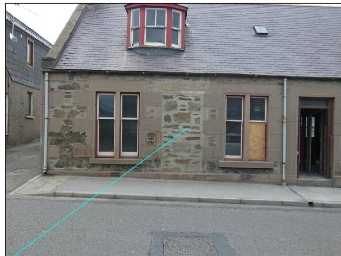
Former Access Door Location
