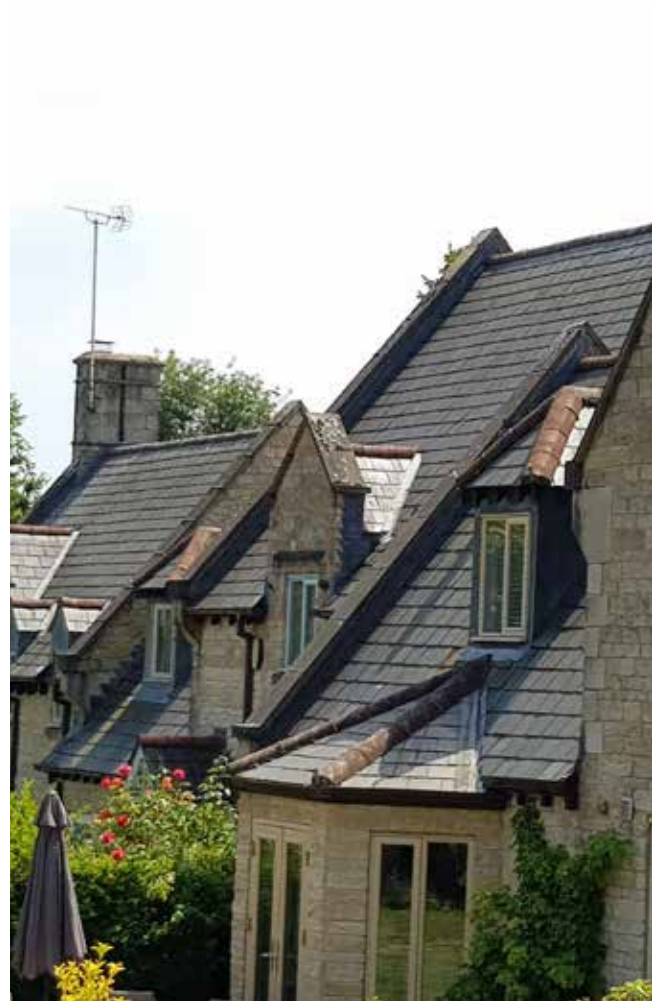
Figure 7: The irregularity of the roofline adds visual interest in the informal and rural character of Barnwell.
