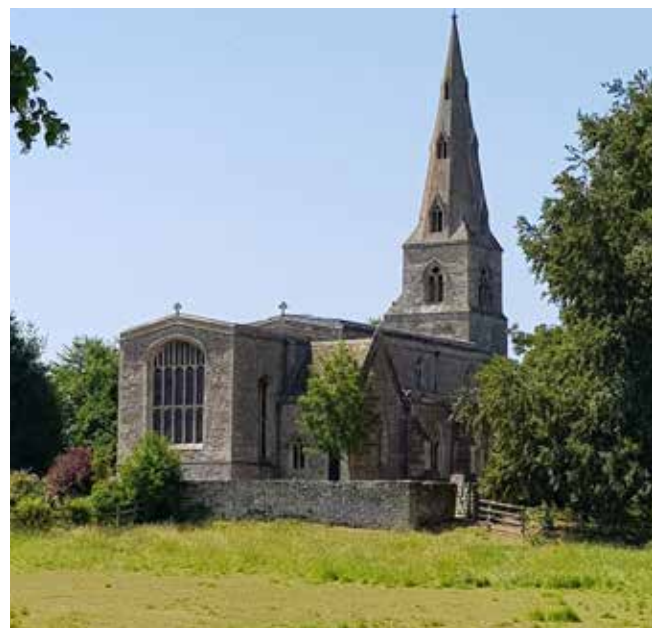
Figure 16: Designated local green space, the Meadow, north of St Andrew's Church.
