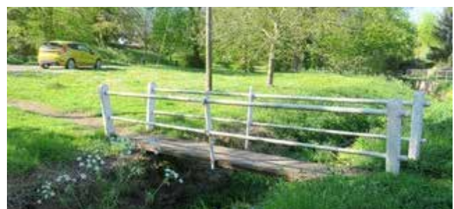
Figure 14: Bridges across Barnwell Brook are a defining characteristic of Barnwell.
