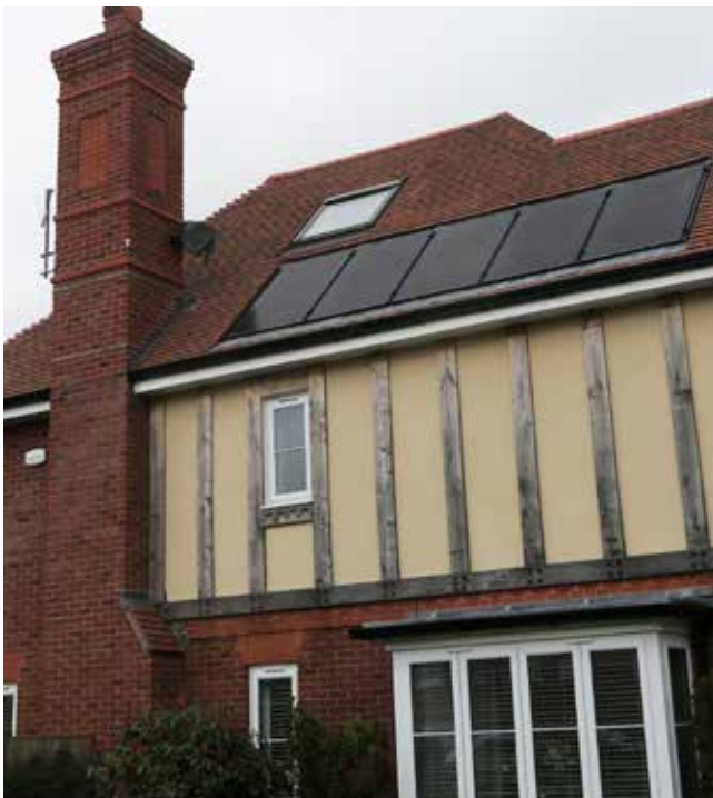
Figure 44: Integration of solar panels on the south-facing pane of the roof of a newly built house.
