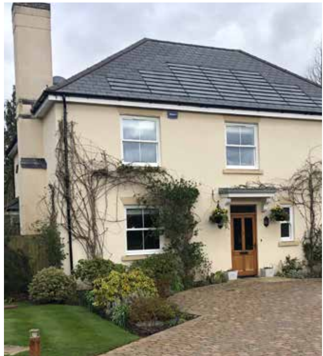
Figure 45: Use of shingle-like solar panels on a slate roof, with the design and colour of the solar panels matching those of the slate tiles.
