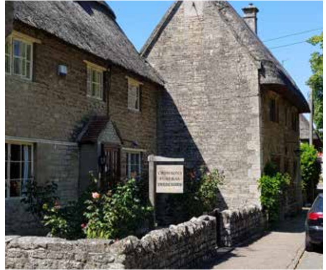
Figure 28: Houses with thatched roofs and casement windows with painted wood lintels. The picture also highlights an informal building line with different recesses and edge treatments.
