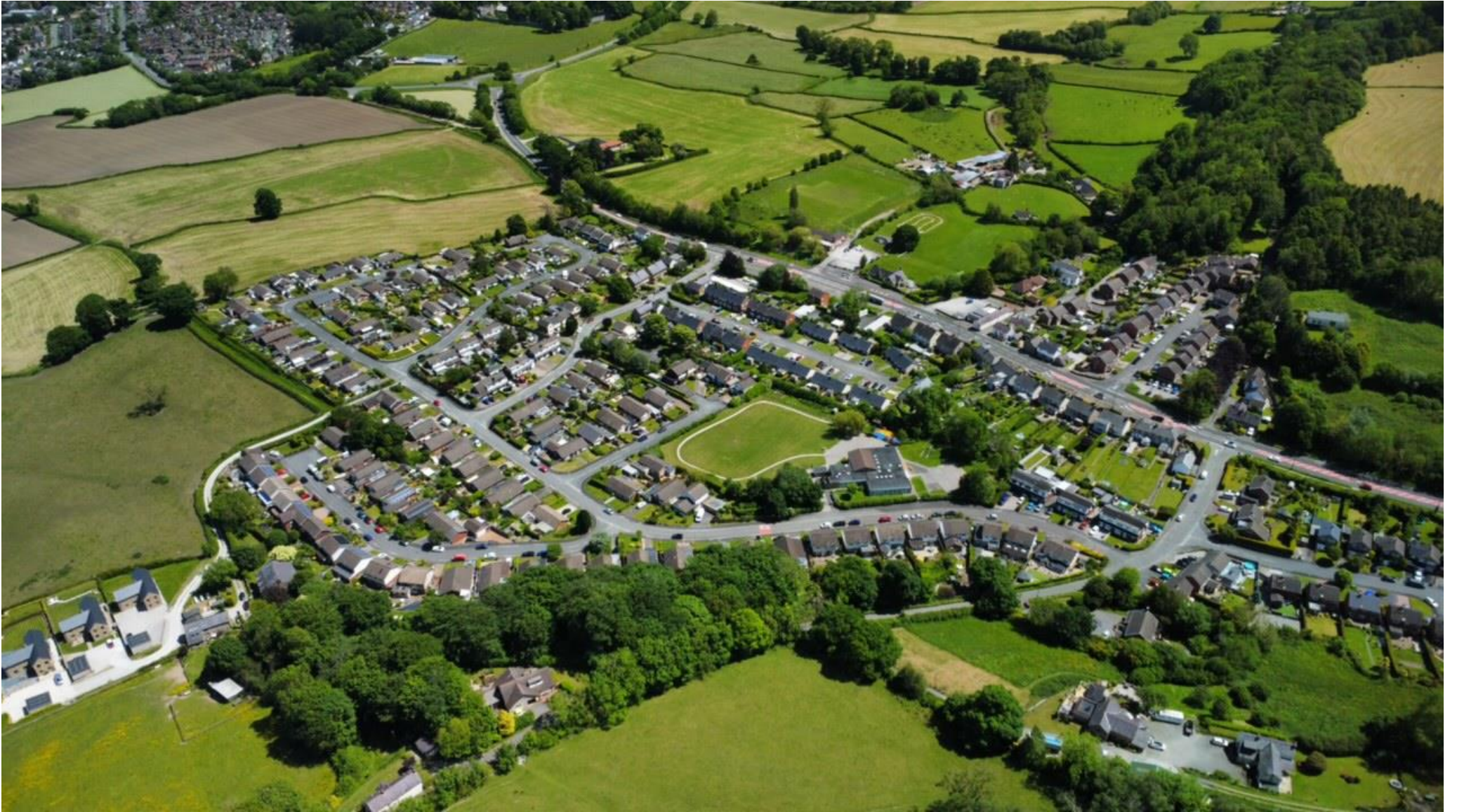
Drone photo of Tros y Wern Estate. June 2024
