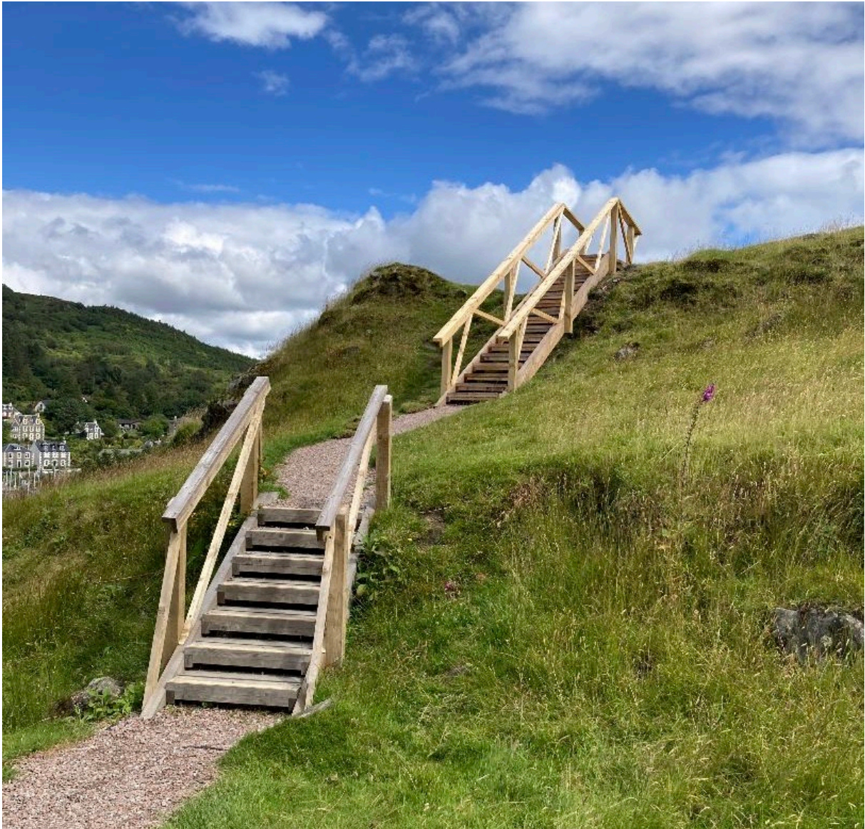
The middle and bottom steps completed
