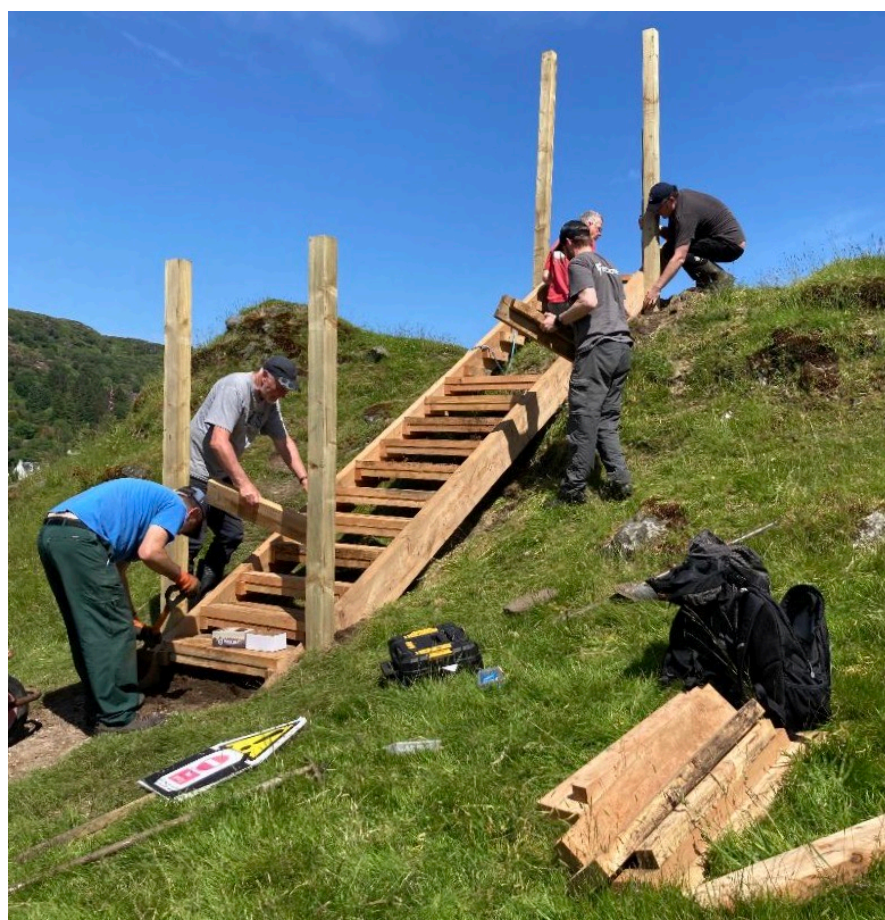
Building the middle steps
