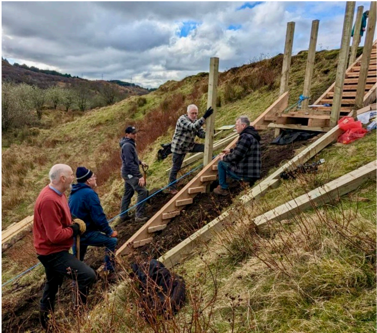
Building the long steps
