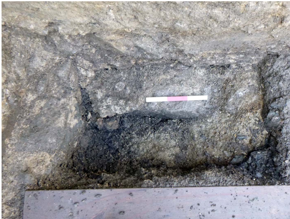
Foundation offset at base of the inner bailey wall
