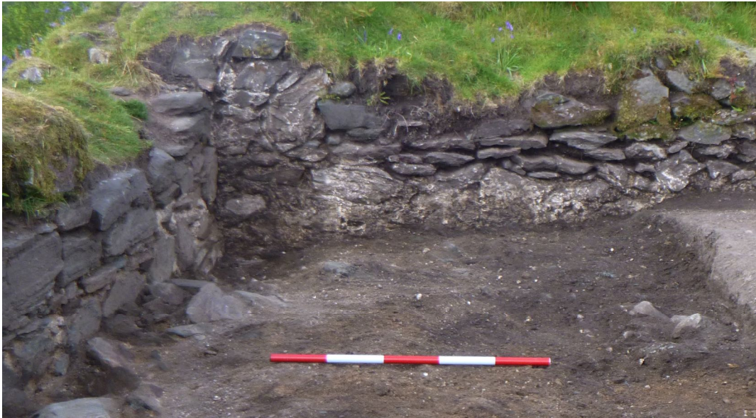
Mortar render on inner bailey wall
