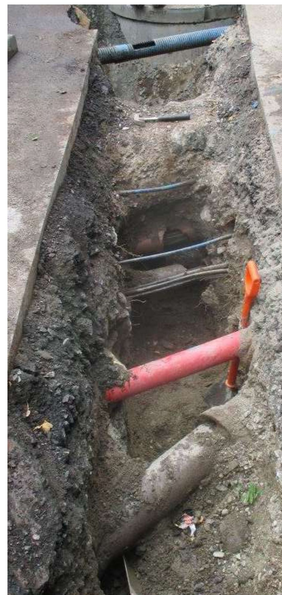
Multiple uncharted services blocking the route to the existing sewer
