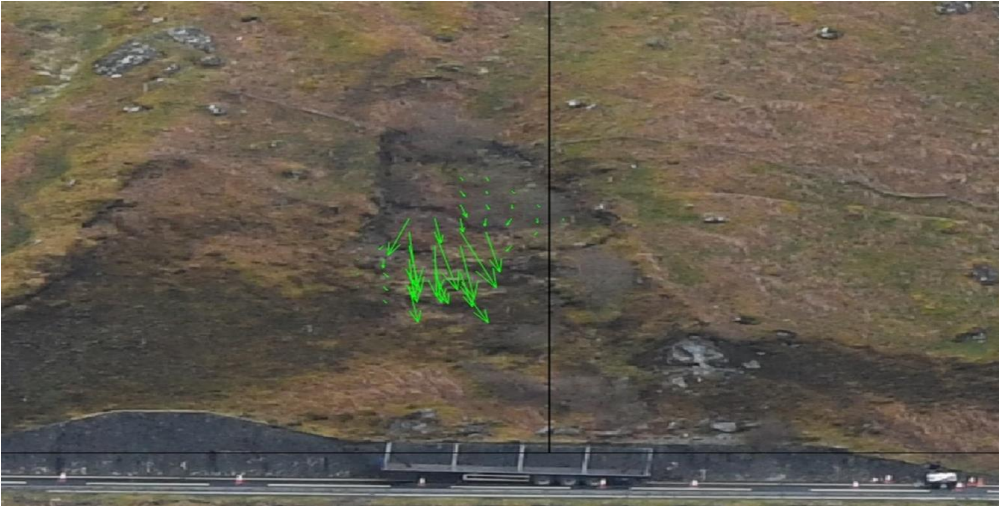
Phase 3a & 3b, Retaining Wall;
