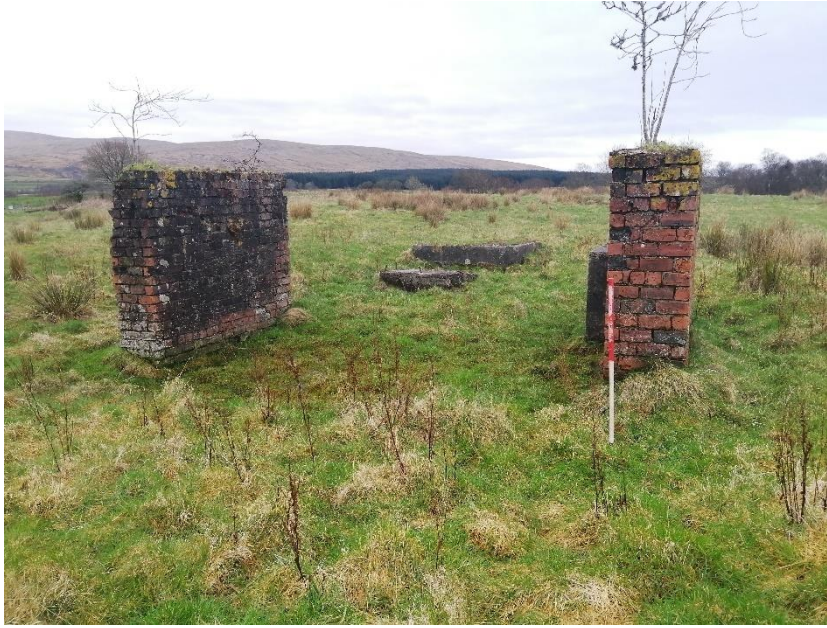
Fig. 9. Site 29, brick built structure
