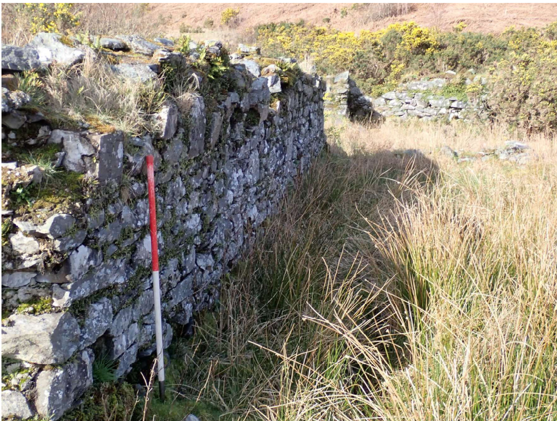
Figure 5: Upstanding wall on the western side of the enclosure (Asset 7).
